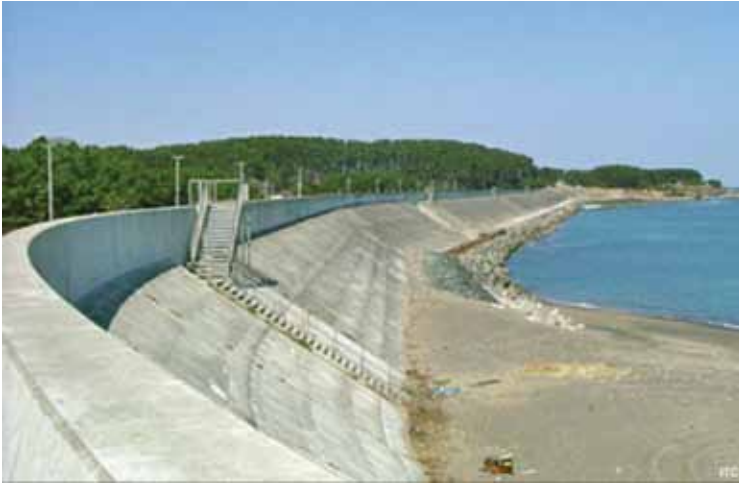
Figure 4.1 Sea wall with stairway evacuation route used to protect a coastal town against tsunami inundation in Japan. Photo courtesy of River Bureau, Ministry of Land, Infrastructure and Transport, Japan.
