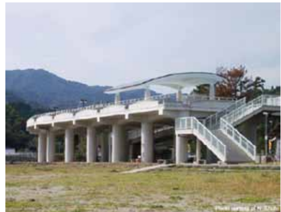
Figure 4.3 Example of an elevated shelter at Shirahama, Tokushima Prefecture, Japan.
